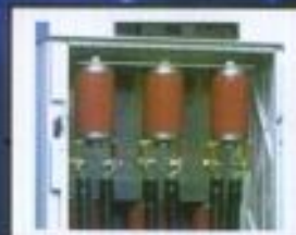
Indoor Surge Arrestor
